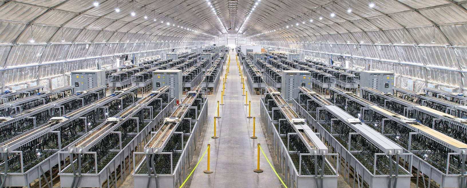
Immersion-cooling bitcoin mining facility in Texas.
